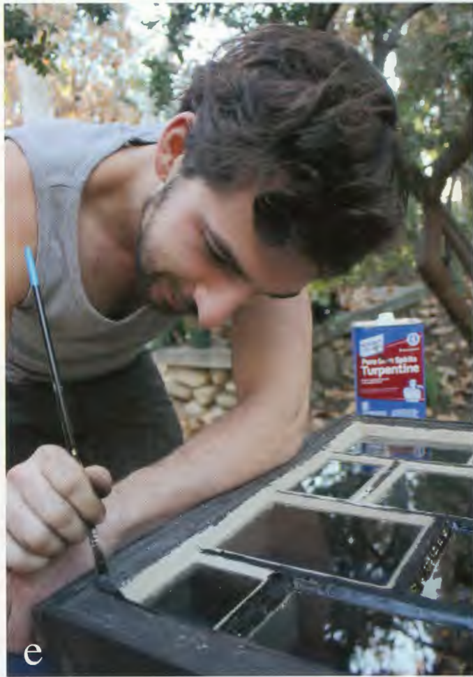
All work performed to Secretary of the Interior's Standard for the Rehabilitation of Historic Buildings . a,b) Original condition of windows casements including deteriorated putty. c) Removal and preservation of original glass. d) Stabilization of carpentry joinery with restoration-grade epoxy and putty. e) Restoration architect, Tada Ryvola, painting windows reglazed with linseed-oil glazing putty to match original finish.
