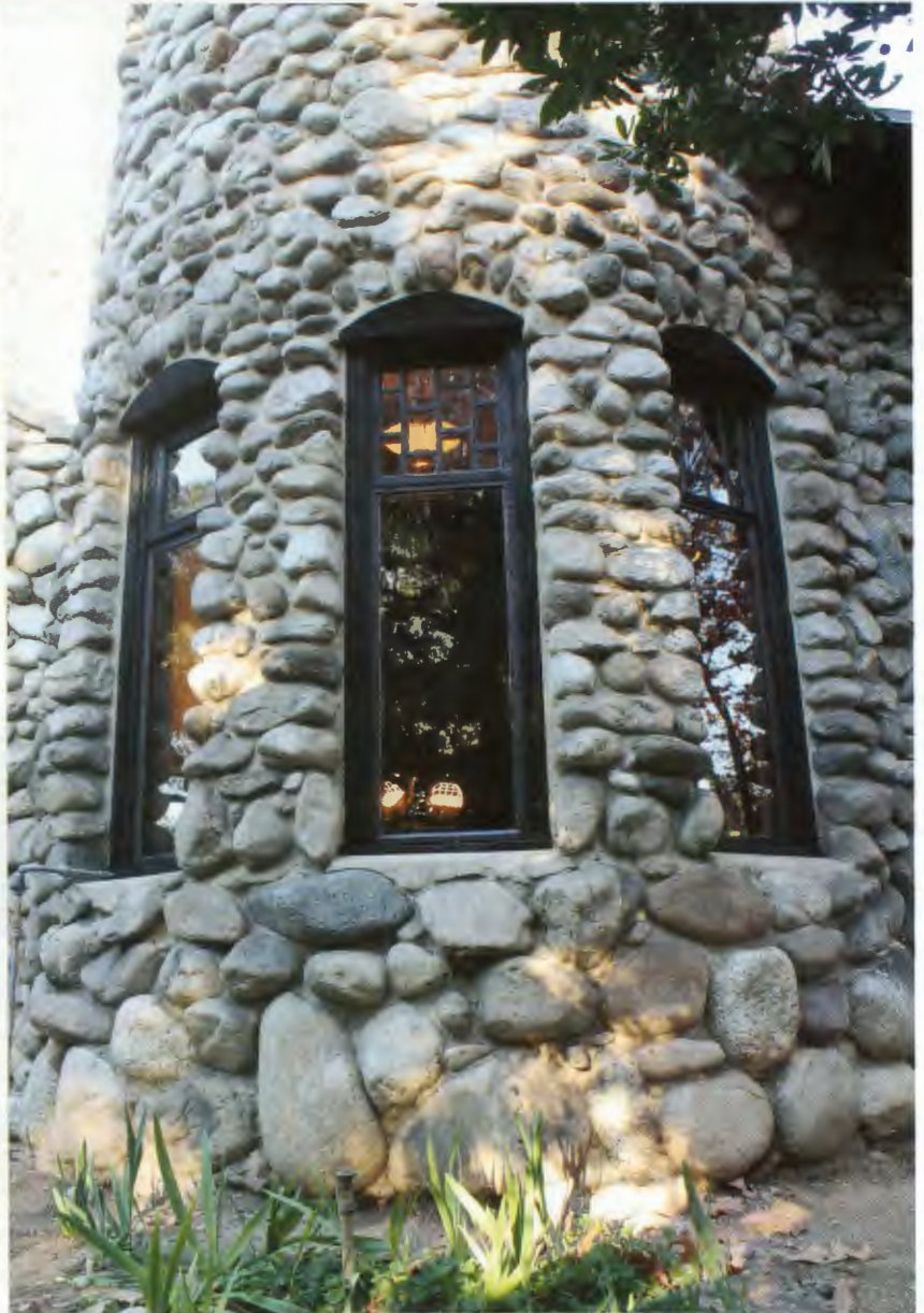
All work performed to Secretary of the Interior's Standard for the Rehabilitation of Historic Buildings . a,b) Original condition of windows casements including deteriorated putty. c) Removal and preservation of original glass. d) Stabilization of carpentry joinery with restoration-grade epoxy and putty. e) Restoration architect, Tada Ryvola, painting windows reglazed with linseed-oil glazing putty to match original finish.
