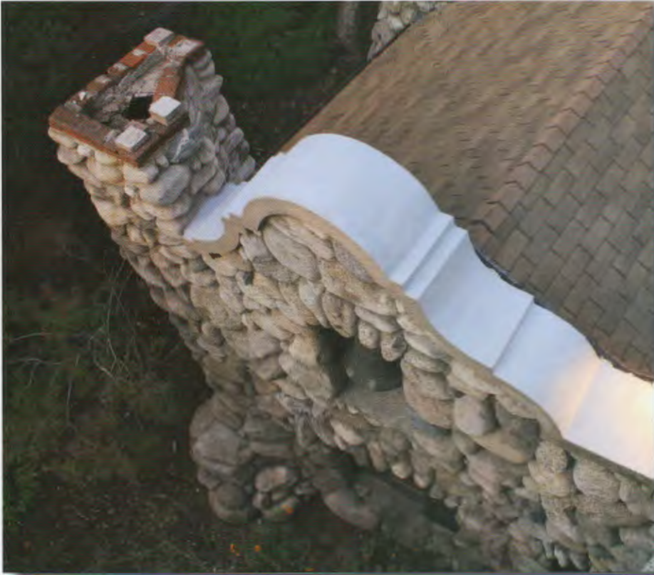
Lummis Home Comedor parapet treated with new sealant.
