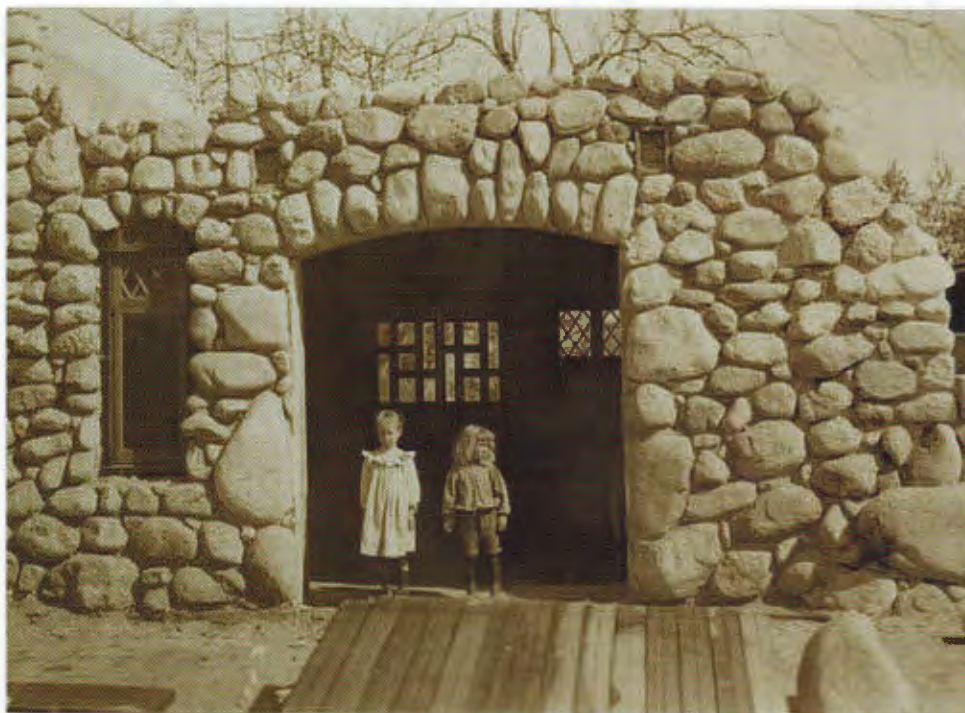
Turbese & Amado Lummis outside Home during construction.
